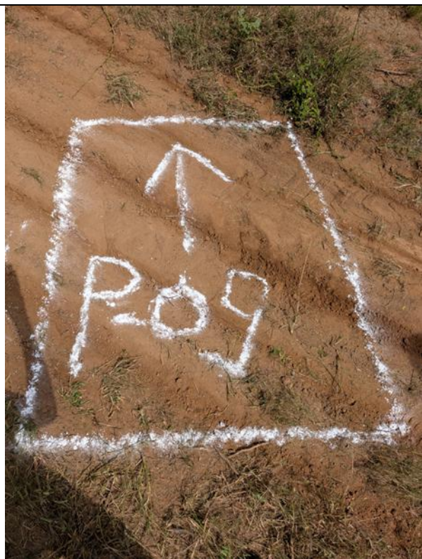
Demarcating the Dimension of Pit
