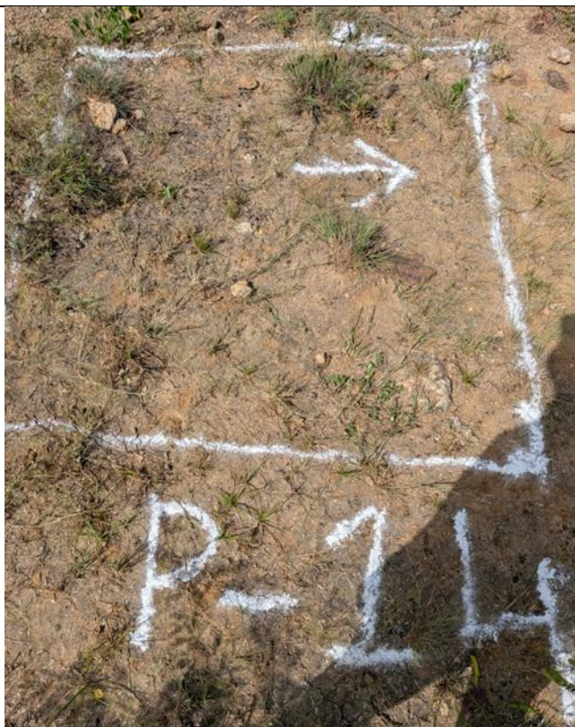
Demarcating the Dimension of Pit
