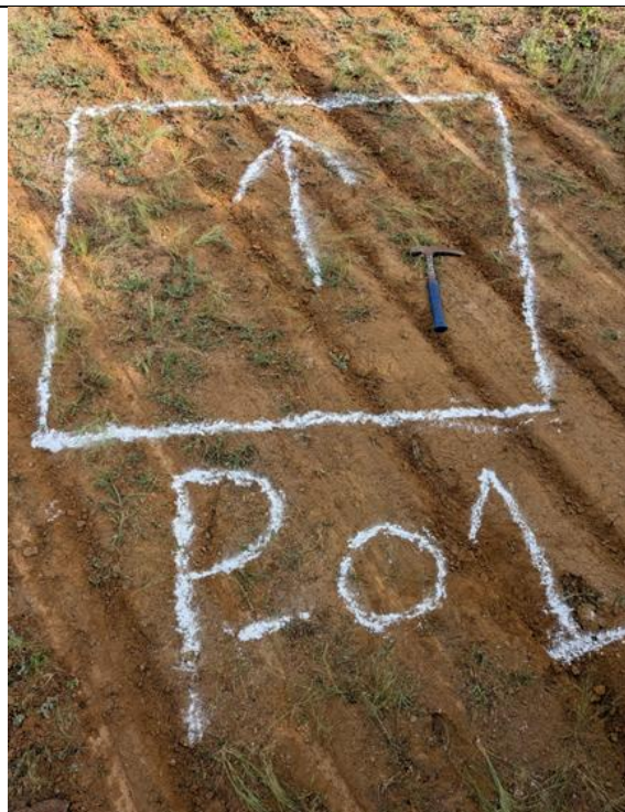
Demarcating the Dimension of Pit
