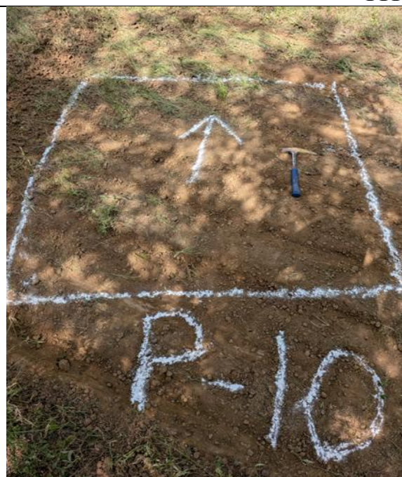
Demarcating the Dimension of Pit
